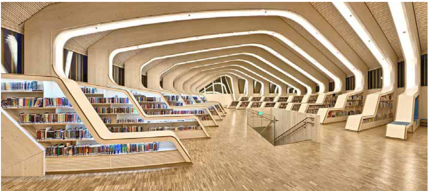
Vennesla Library in Norway. Interior supportive glulam beam system treated with clear water based flame retardant coating to B s1 d0.
